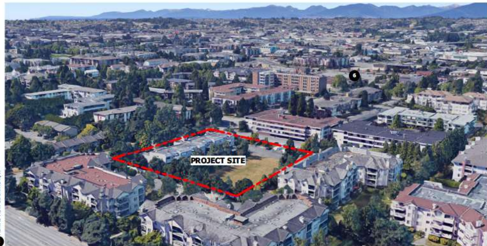
8 AERIAL VIEW LOOKING NW
