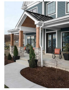
WOOD COLUMNS W/ STONE BASE
