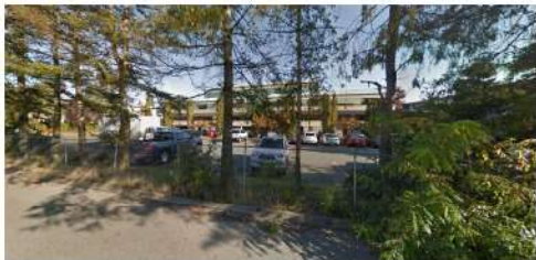
existing building looking north
