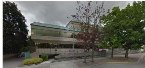
existing building looking south
