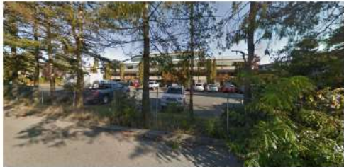
existing building looking north
