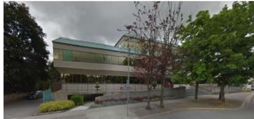
existing building looking south
