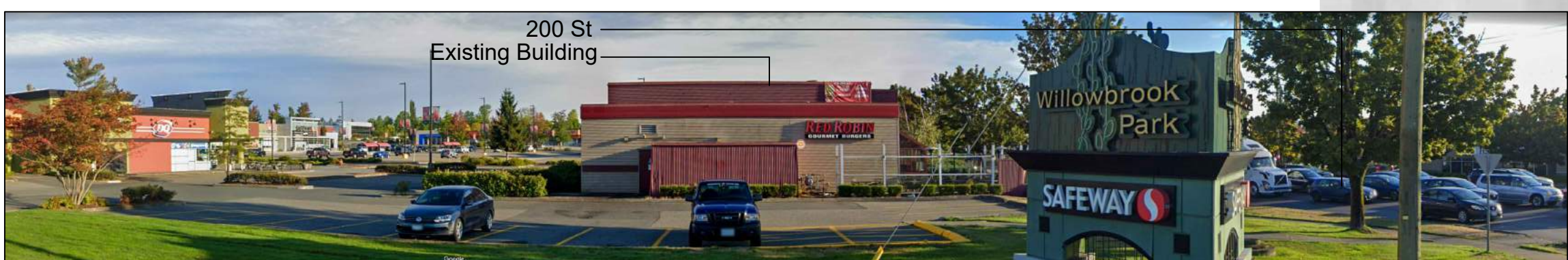
4 Existing Building from Langley Bypass (South Elevation) NTS
