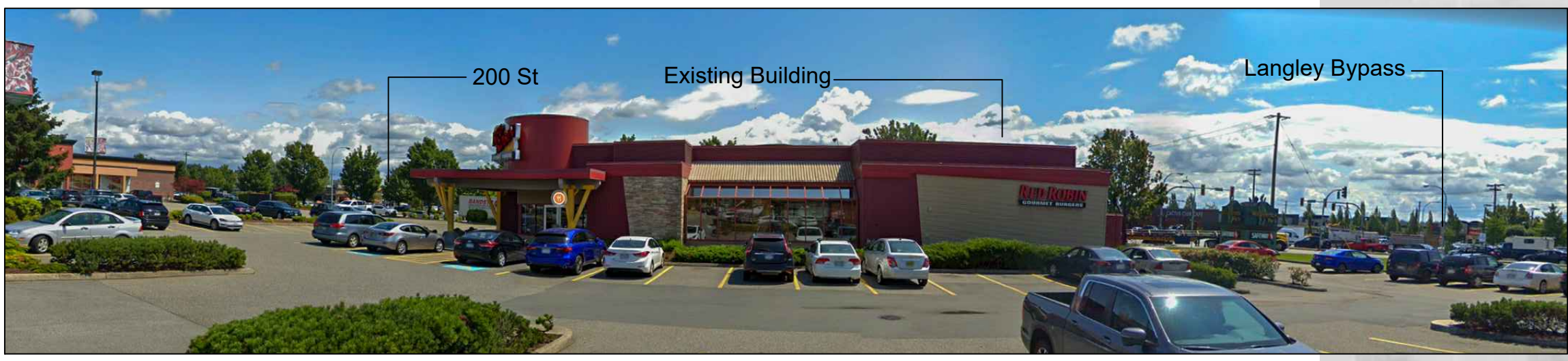
3 Existing Building from parking (West Elevation) NTS
