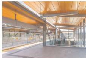
Coquitlam Central Station
