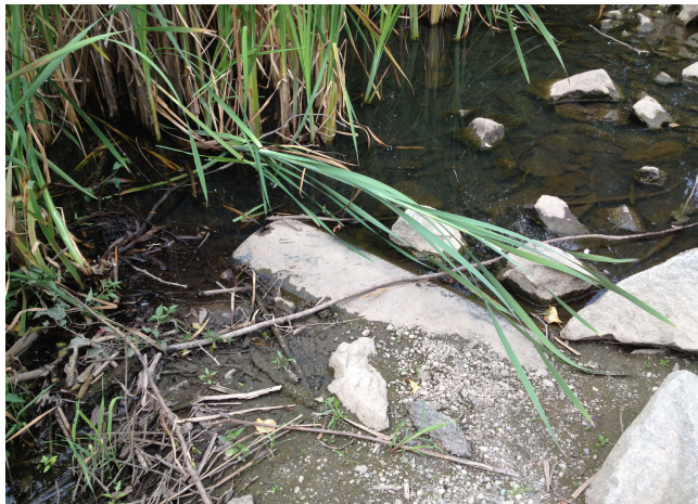
3 Pond Outlet Culvert to Nicomekl River
