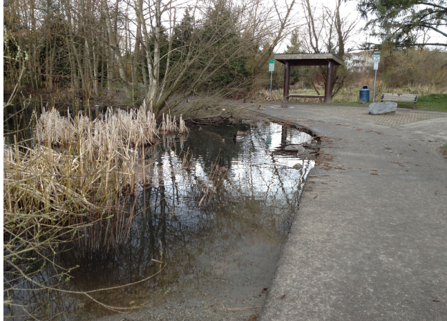
4 High Water Level in Pond
