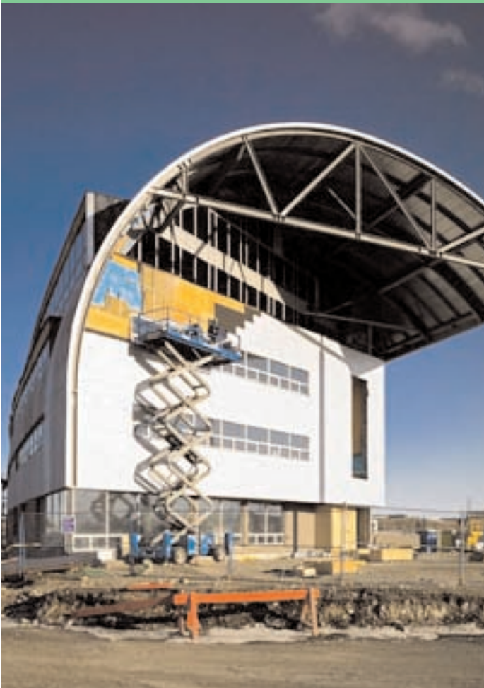
The Water Centre revitalization project in Calgary.
