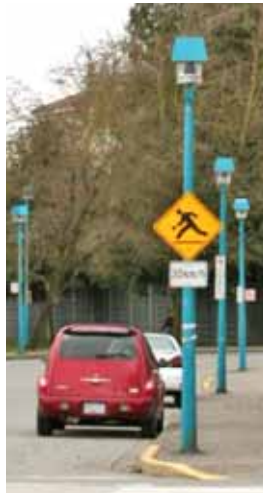
existing Carriage lights
