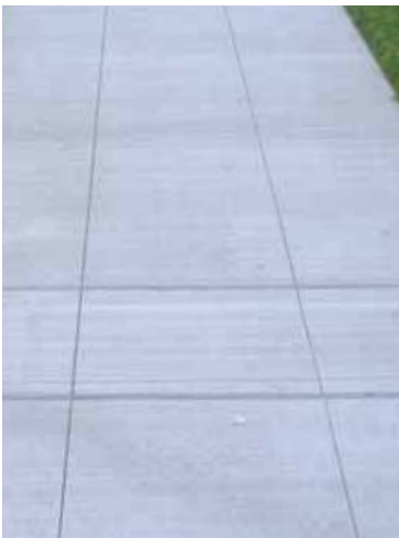
CIP Concrete Sidewalk
