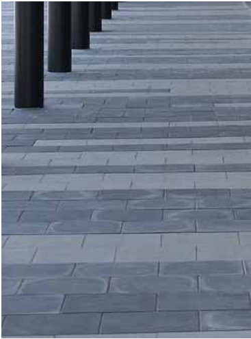
Concrete Unit Paving
