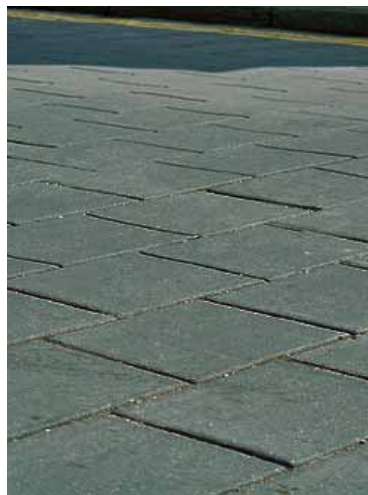
Concrete Unit Paving
