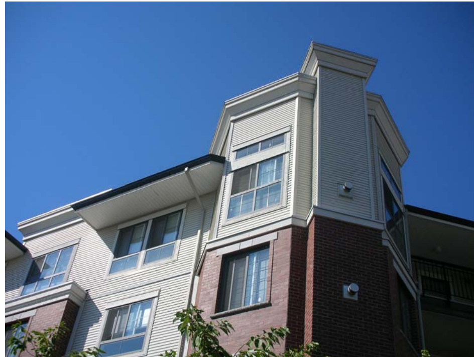
High quality exterior finishes and materials
