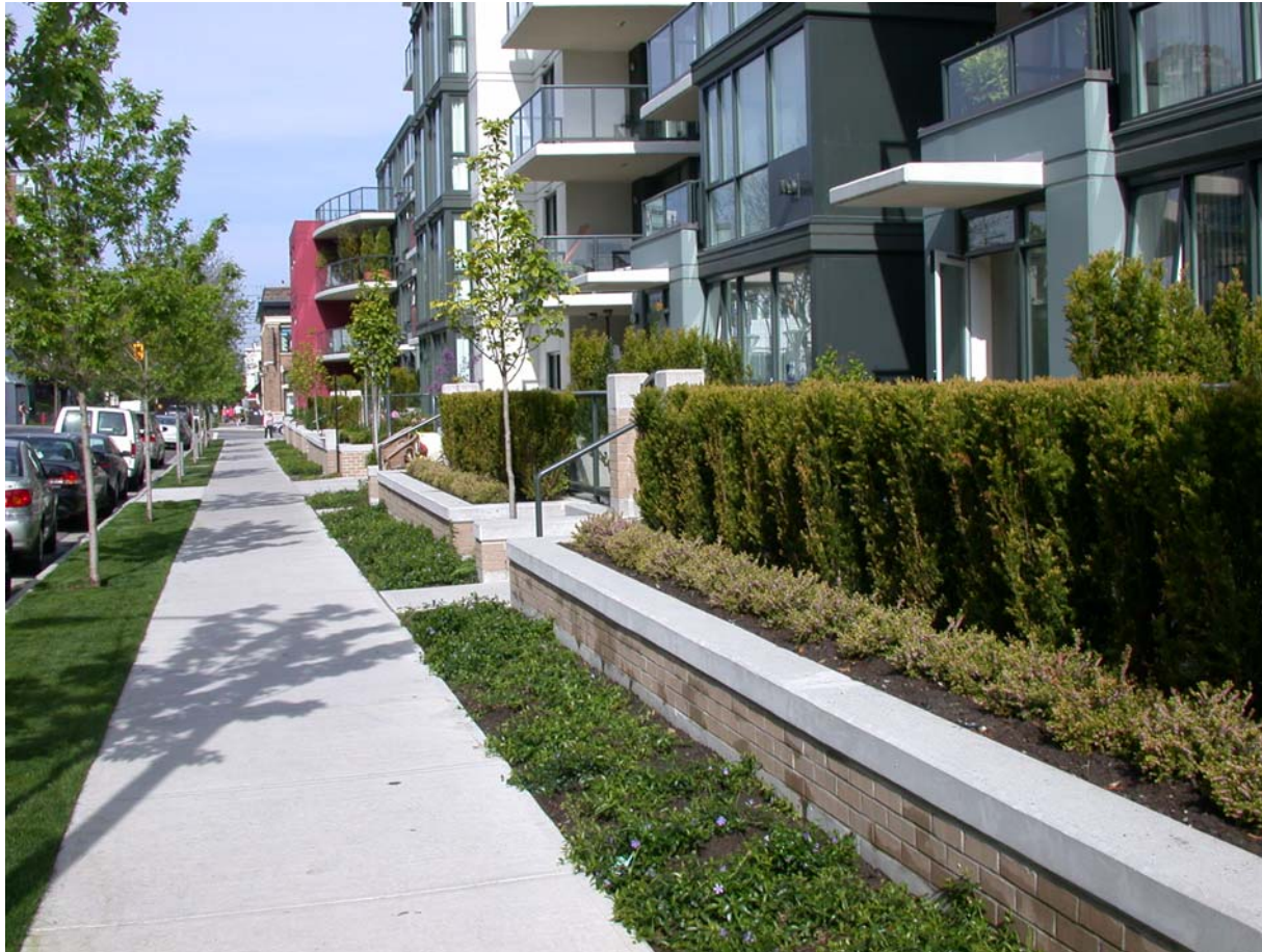
Attractive street-oriented development
